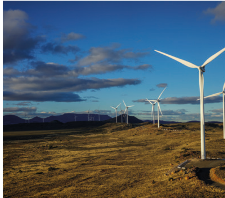
The 27MW Metrowind facility, in South Africa's Eastern Cape Province
